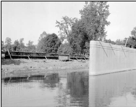
Historic bridge pier in the water. (MDOT)
