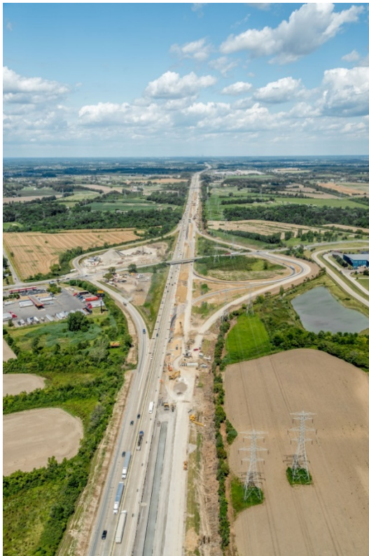
Aerial view of I-75 reconstruction.
