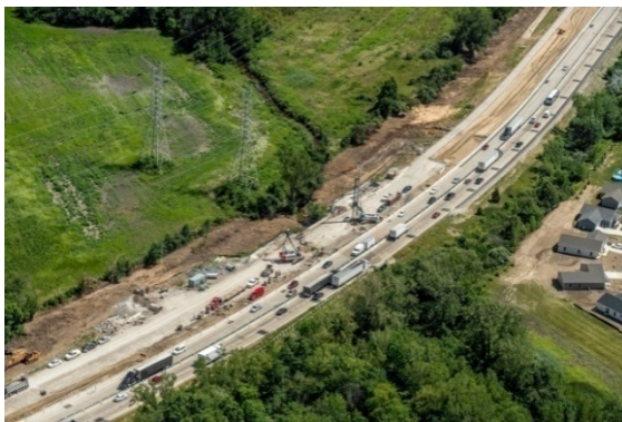
Northbound reconstruction on I-75.
