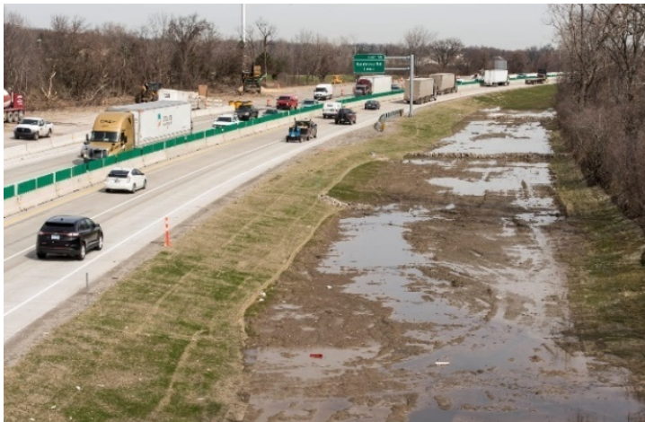
Wide grassy swale helps reduce runoff and improve water quality on the 2015 construction segment.
