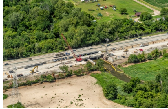
I-75 construction in Monroe County, 2015. (MDOT)
