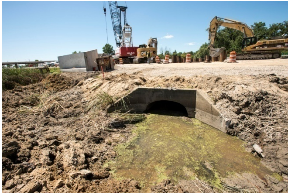
(Left) Outdated culvert on I-75 before reconstruction. (Right) A large box culvert replacing a twin culvert, I-75, Summer 2015.
