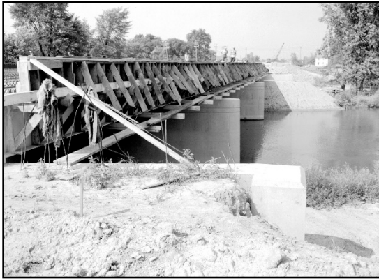
Historic construction of a bridge. (MDOT)
