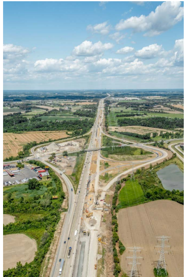
Aerial view of I-75 reconstruction.
