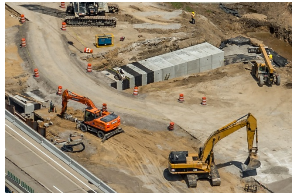
(Left) Outdated culvert on I-75 before reconstruction. (Right) A large box culvert replacing a twin culvert, I-75, Summer 2015.
